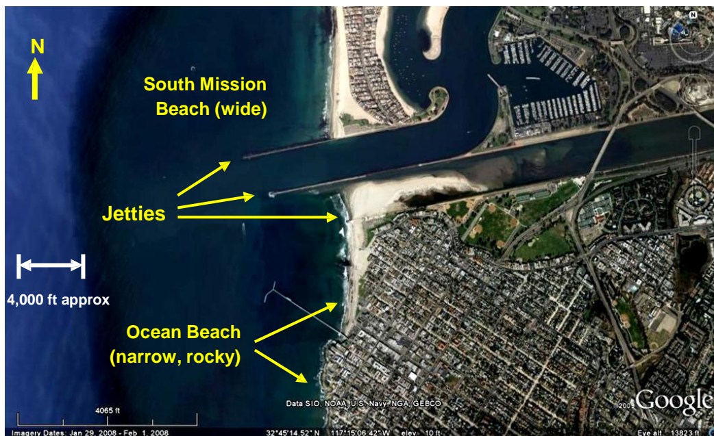
Mission Bay jetties, San Diego, CA (image courtesy of Google Earth)
